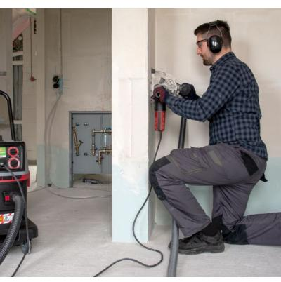
What kind of safety vacuum cleaner is suitable for your application? The dust classes provide the answer to this question. Materials and their dusts are classified according to them and machines are certified, because the vacuum cleaners meet the corresponding require-
