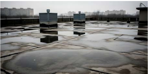
flat roof renovation
