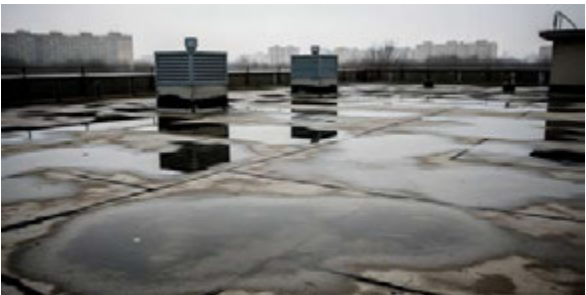
flat roof renovation
